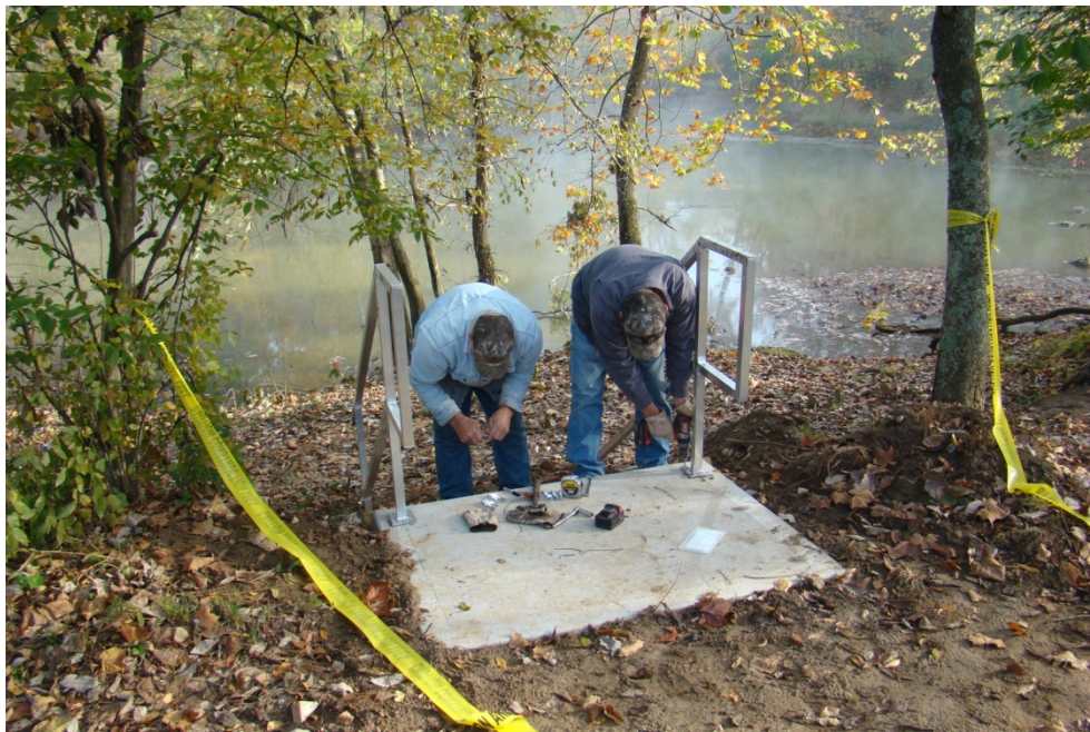
Contractor installing hand railing on Access #2
