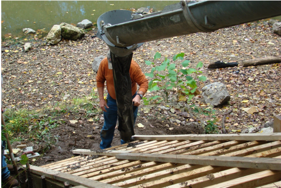
Concrete begins to flow for steps at access #1
