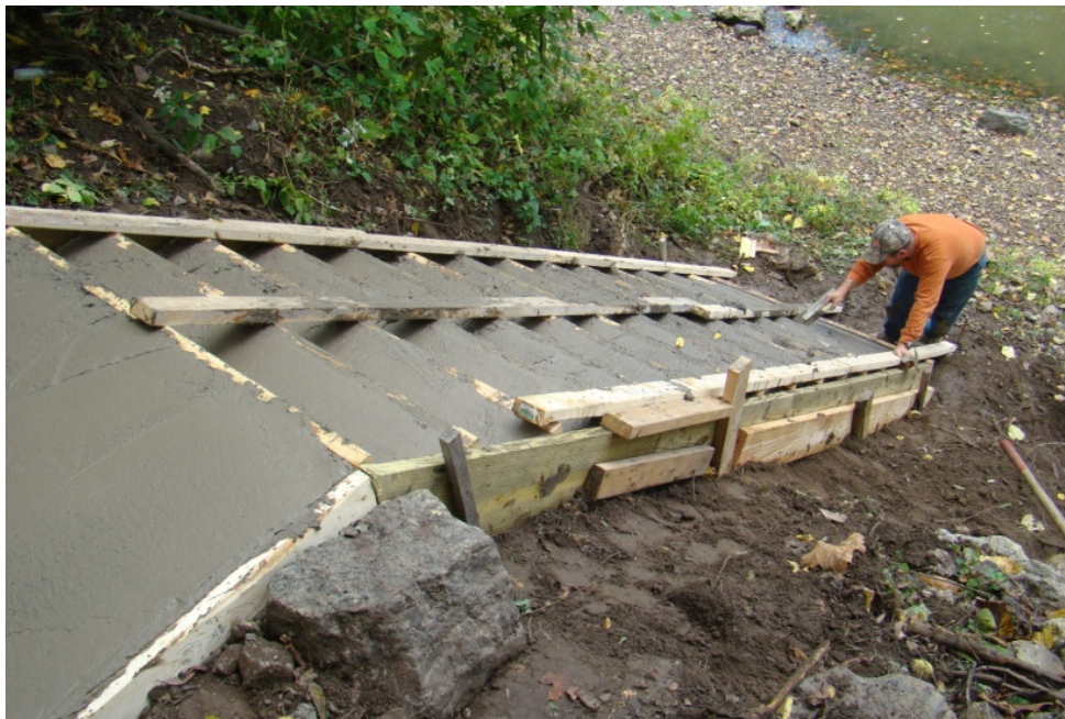
Access #1 First concrete pour, contractor at work leveling
